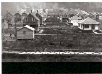
Company homes near Fraser Mills. Sidewalks were made of wood so they would float during spring floods.
